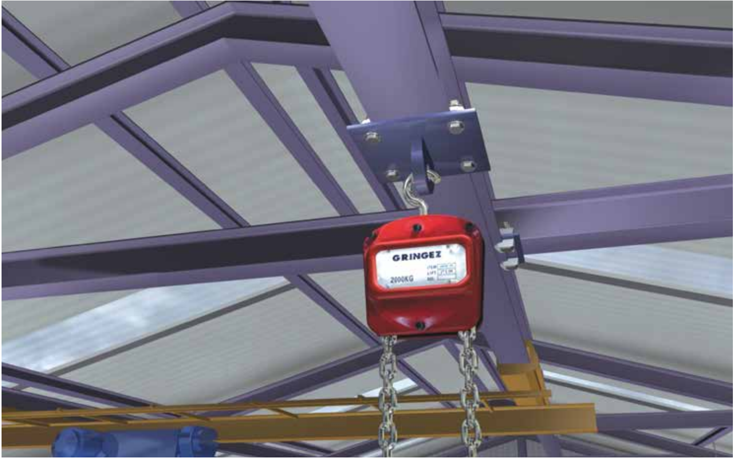
Installation of lifting equipment
